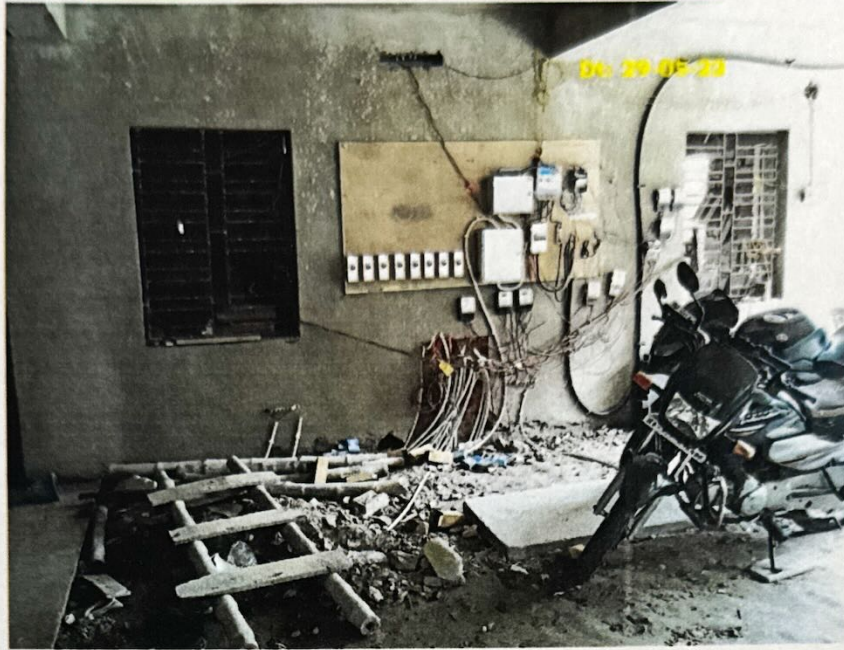
GROUND FLOOR STATUS as on 29-5 -22
